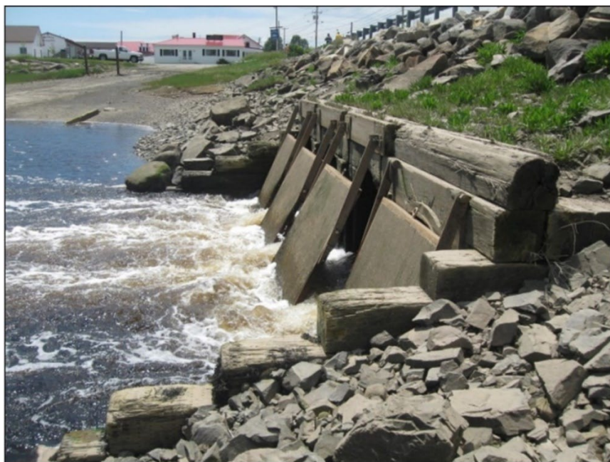
Figure 2: Seaward Culverts with Flap Gates during Low Tide
