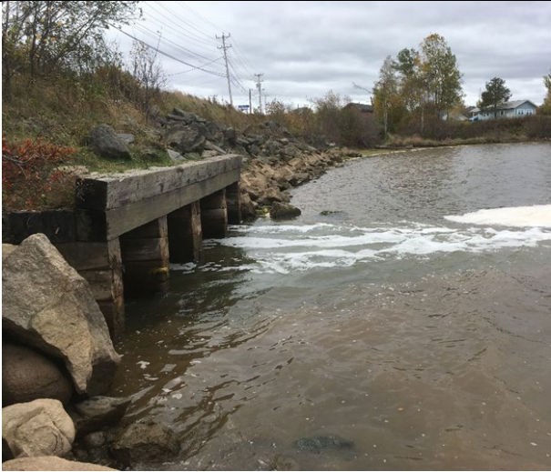
Photo 1. Middle River box culvert and riprap shoreline during rising tide
